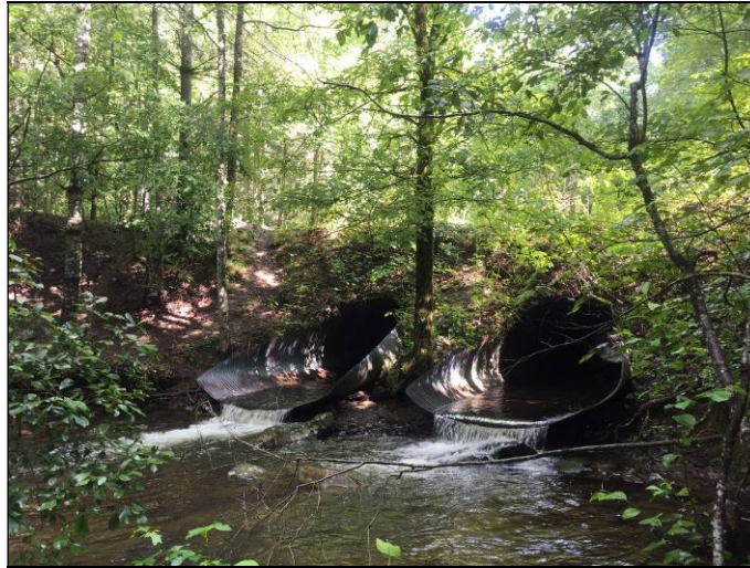
Fig. 1. Baseline: Two perched culverts, with the one on the right collapsed in the center. By the time we started construction the collapse had blocked all flow through that culvert and there was significant scour downstream.
