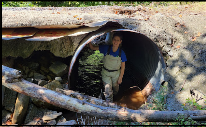
Surveying a failing culvert in the Holly Creek watershed
