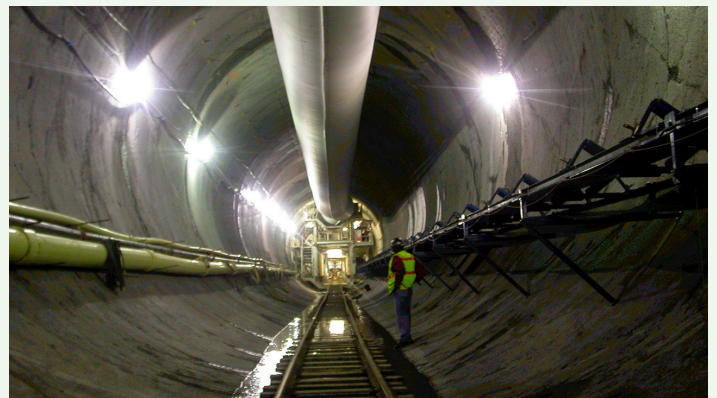
West Combined CSO Storage Tunnel, Atlanta, GA
